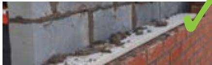
**Do** keep the top edges of the insulation clean of mortar by using a cavity board.
