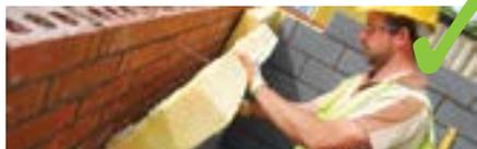
**Do** stagger vertical joints and ensure they are tightly butted.
