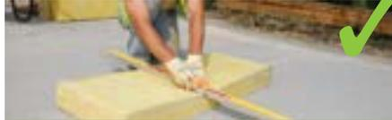
**Do** cut the insulation using a sharp knife and straight edge.
