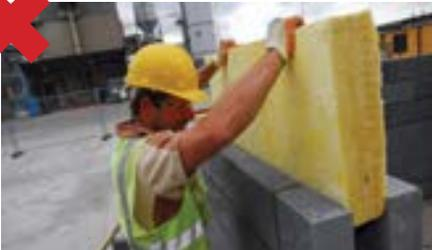
**Do not** push insulation down into the cavity as a tightly butted horizontal joint cannot be ensured.
