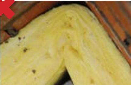
**Do not** bend insulation around corners as this creates air pockets within the cavity.
