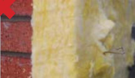
**Do not** pierce the insulation with wall ties to prevent tearing the insulation, creating a potential thermal bridge.
